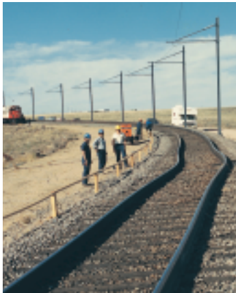
FIGURE 13–17 The extreme temperatures of a July day caused these railroad tracks to buckle.
